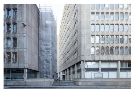
The current office building stands out due to its striking S shape and rhythmically constructed façade comprising prefabricated concrete units.
